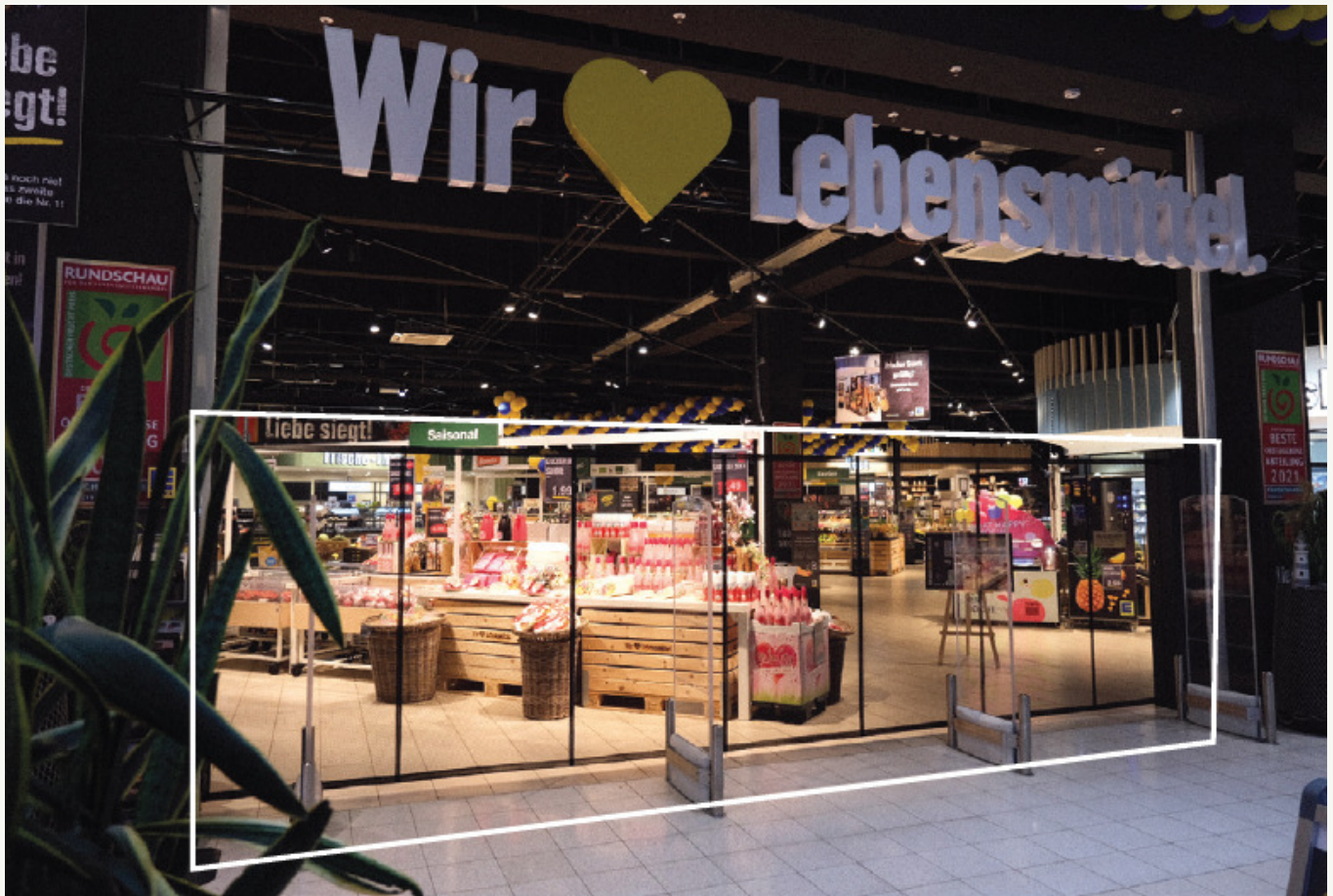
Installed at a store entrance · partition area outlined in white
